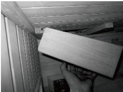
FIG 15.2 Installing the Radio Wood Housing
