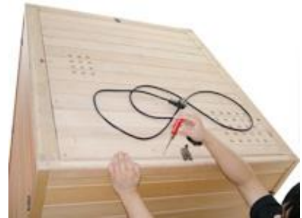
FIG-18 Screw down the Roof Cover
