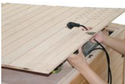
FIG 17 Slip the power cord through Roof Cover
