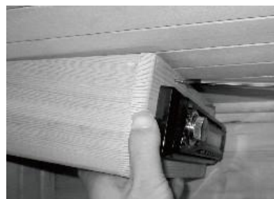
FIG 15.3 Screwing in the Radio Wood Housing
