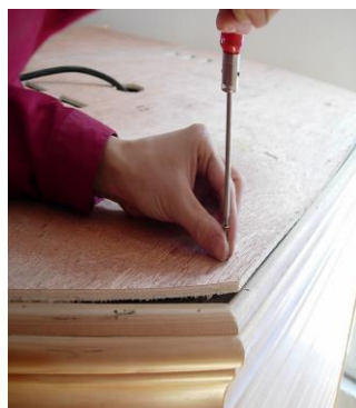
FIG 18.1 Screw down Roof Cover
