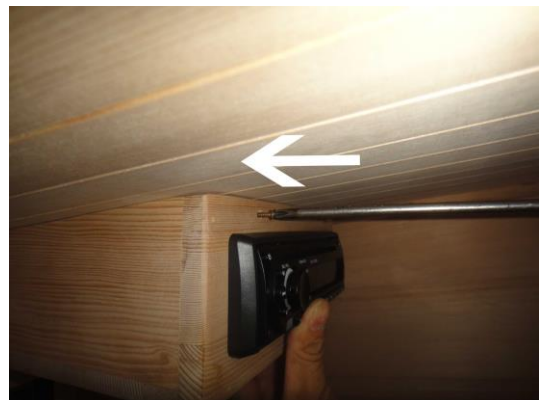
FIG 15.4 Screw wood housing to sauna room
