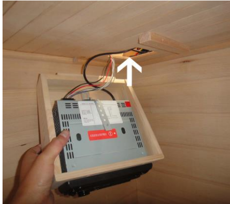
FIG 15.3 Feed the wires up through the roof
