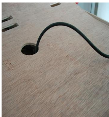
FIG 18 Pull Power Cord through Roof Cover
