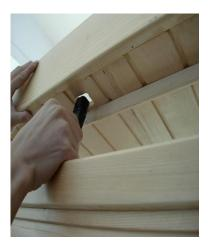
FIG-13 Slip cords/wires through corresponding holes
